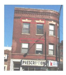
We will re-point and replace damaged bricks in the area marked on the image. The cracked window sill will be removed, glued with epoxy and reset back.
