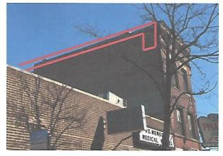
The chimney shown on the image will be rebuilt to the roof level, the flue liners will be replaced if necessary and the new concrete cap will be installed on the top of the chimney.
